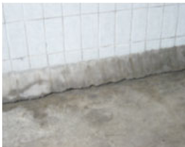
Fig. 474: Proper cleaning/sanitation not possible. Crack in junction wall/floor
