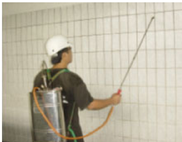
Fig. 493: Disinfection of walls by using portable spray equipment. For operator's protection gloves and facemask are recommended.
