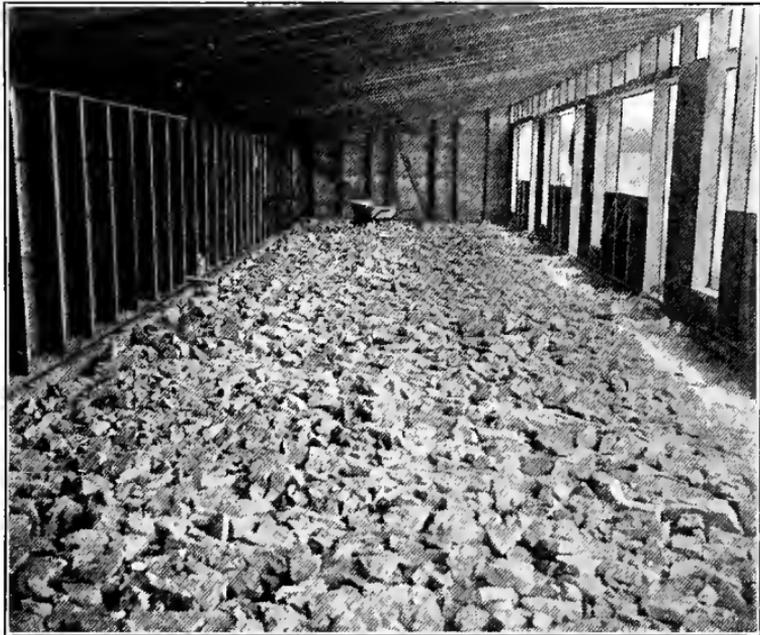
A six- or eight-inch course of coarse crushed rock should be the floor foundation. (Courtesy of Kansas Experiment Station.)
