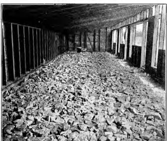
A six- or eight-inch course of coarse crushed rock should be the floor foundation. (Courtesy of Kansas Experiment Station.)
