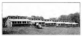
A row of half-monitor roof fresh-air houses. (Courtesy of F. L. Sewell.)
