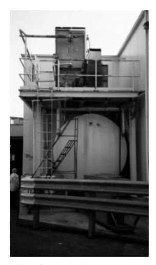
**Fig. 10.9** Water prerequisite – cooling water reservoir.
