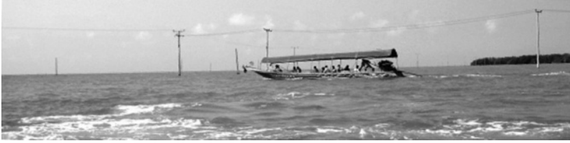
FIGURE 5 A line of telegraph poles south of Bangkok, Thailand: built on subsiding land, they are now up to 1 km out to sea.
